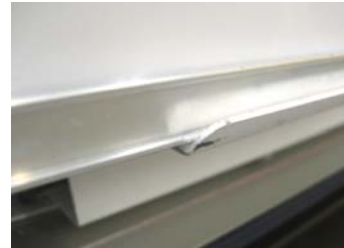
Lower diffuser panel onto shelf
