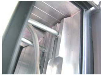
Slide T-pins up into extrusion slots
