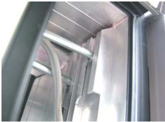
Diffuser panel in position
